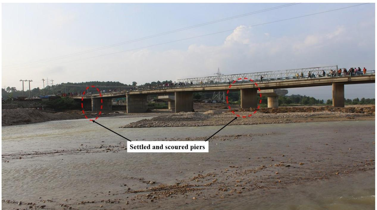
*Fig. 3 Ratu bridge damaged due to settlement and scouring in Mahottari district*
