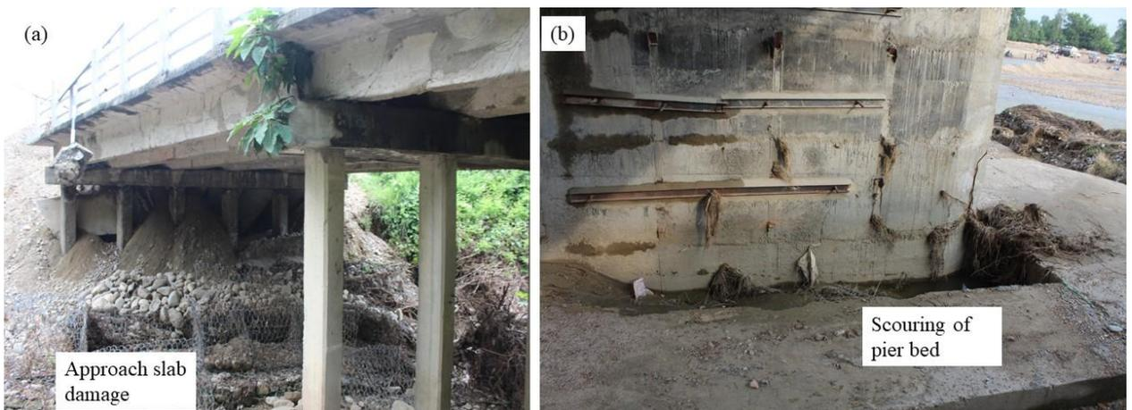
*Fig. 5 a) Approach slab damage due to the flood, b) scouring of pier bed*
