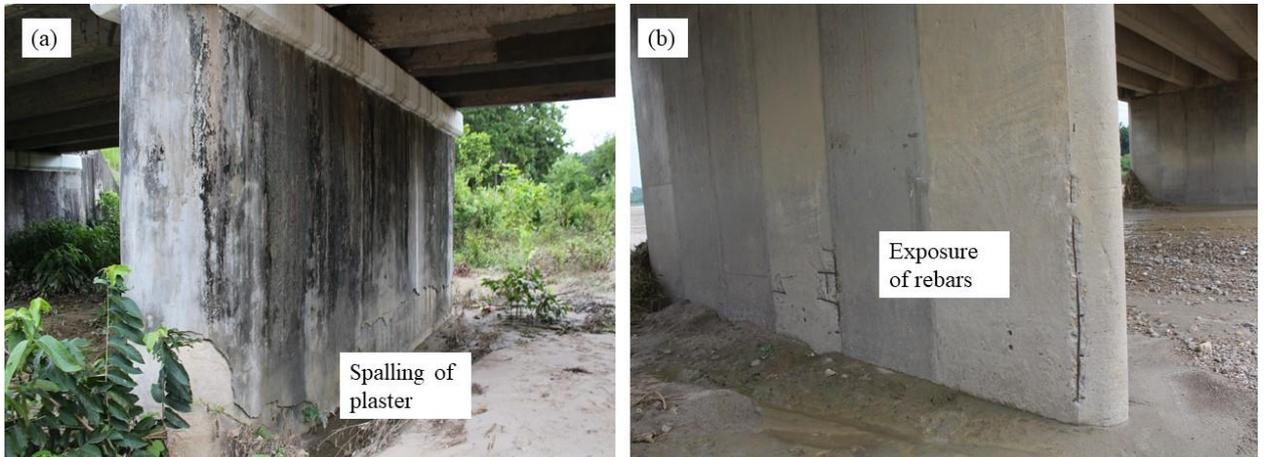
*Fig. 4 a) Spalling of plaster due to 2017 flood, b) exposed re-rebar due to flooding*
