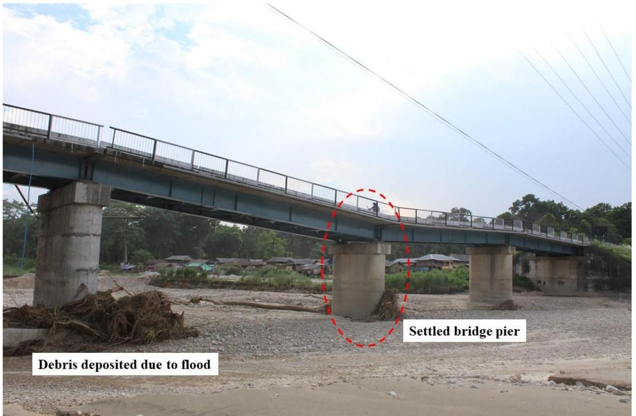
*Fig. 2 Dudhaura bridge damaged due to settlement and scouring in Bara district*
